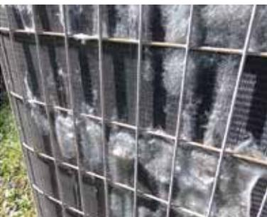
This can lead to overheating of mechanical components (like the compressor), impacting the efficiency of the A/C, increasing cooling costs and can even cause the system to completely fail.
